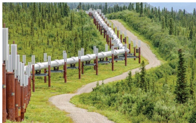
The Alaska Pipeline.
